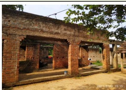
Incomplete Kitchen-cum- dining room at CCI, Mangalpur
