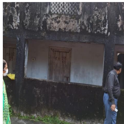
Outer condition of the first floor
