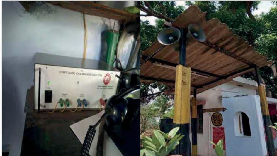
Figure 2.23: SR: Honey Bee Sound Device equipment installed at LC No. 154 (A line) between Walayar and Kanjikode
