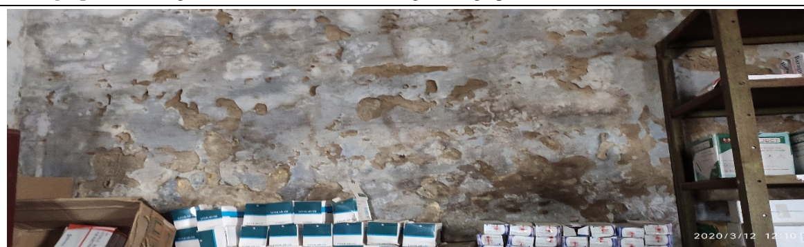
Photograph 5.6: Seepage in an entire wall of storeroom where medicines are stored in DH Kohima
