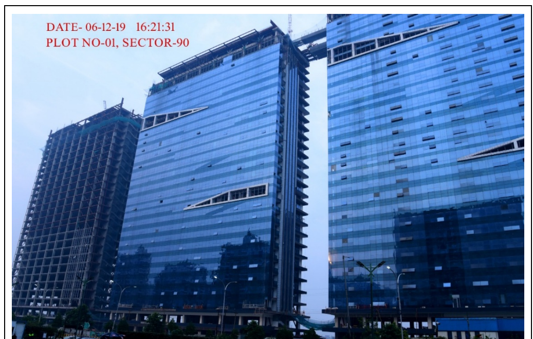
Photograph 5.4.6: Status of construction on Plot No. 1 in Sector 90
