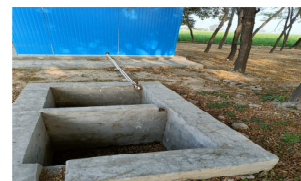
Disposal of water of RO plant at Shergarh (Fatehgarh Sahib) 21.12.2021
