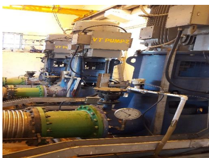
Pump House of Amath Mega Lift Project
