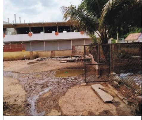
Picture No. 6.3.6: Water logging at Harihara bus station (June 2019).
