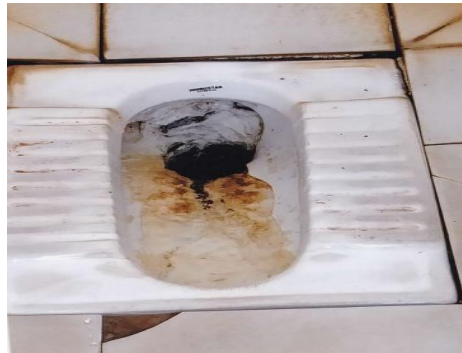
Picture No. 6.3.7: Srinivasapura old bus station - Damaged toilet (April 2019).
