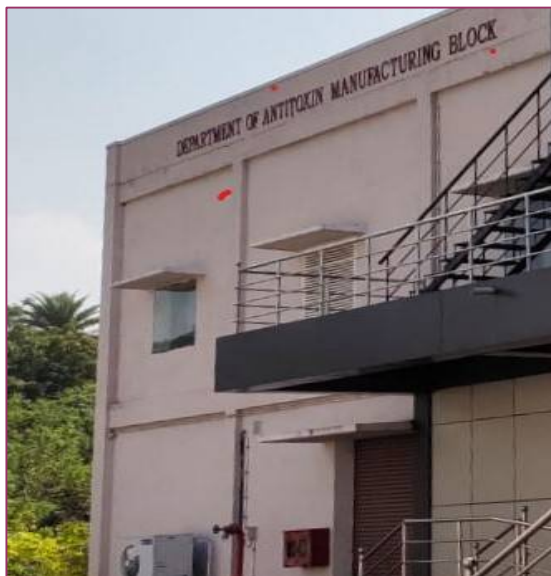
Exhibit 3.1: Newly constructed DAT building
