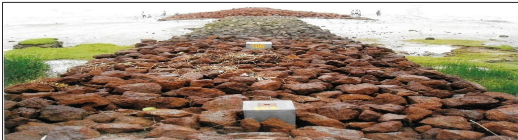
Image 6.1 Construction of spur
