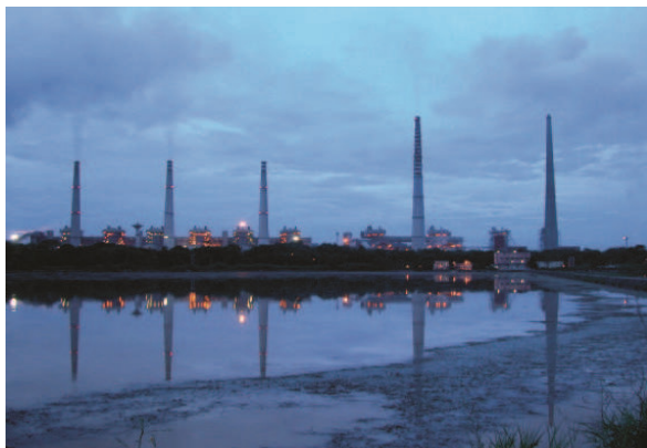
Picture 8: Ash Pond of Captive Power Plant at Angul
