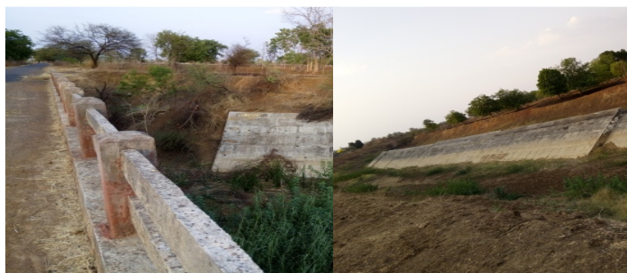
Skidding of Retaining wall at RD 31020 m
