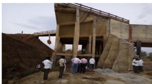
Repair work of aqueduct on Down Stream side under progress
