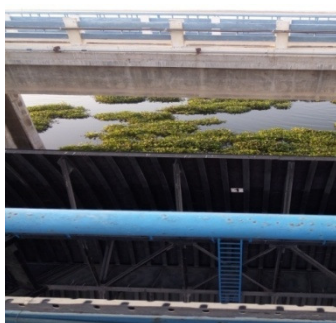
Echhornia Plant growth in front of gate number 3 of the Gosikhurd Reservoir
