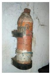
Picture 6.1: Poorly maintained fire extinguishers in Brilliant Ice Plant, West Hill, Kozhikode (18 May 2017)
