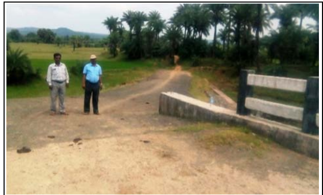
Bridge over Chhotalaxmi Nala between Chhotalaxmi and Basaha Mission with no approach road
