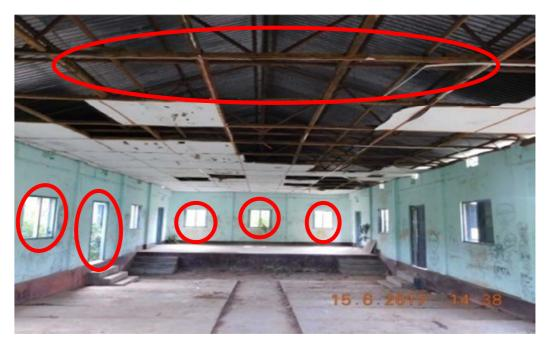
Photograph 4.3.11: Dilapidated condition of the community hall with broken doors, windows and ceiling
