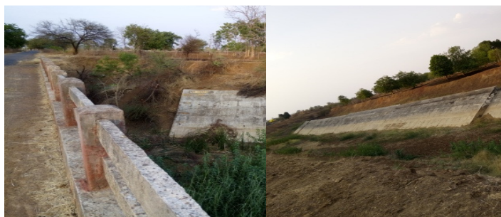
Skidding of Retaining wall at RD 31020 m
