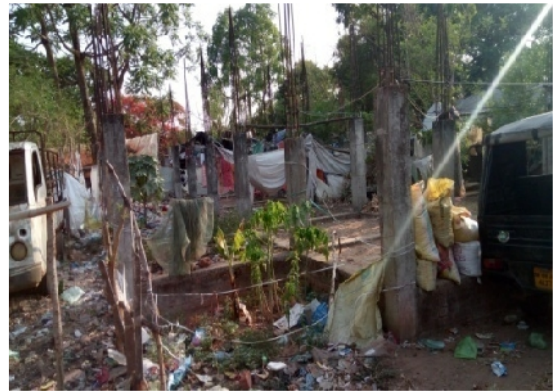
View of abandoned night shelter at Jobra, Cuttack
