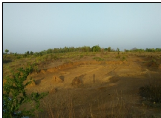
Renovation of Balpall Tank in Chhakarmal GP of Sonapur PS
