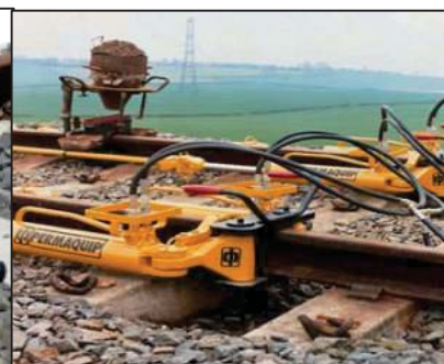
Figure 10: Rail Creep Adjuster
