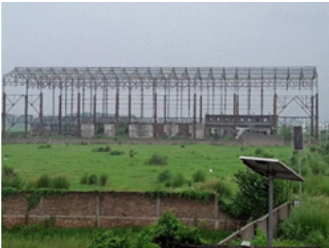
Figure 3.2: Incomplete Raw materials Processing Facility
