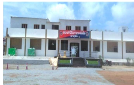
Stadium at Suryapet occupied by Police Department (June 2017)
