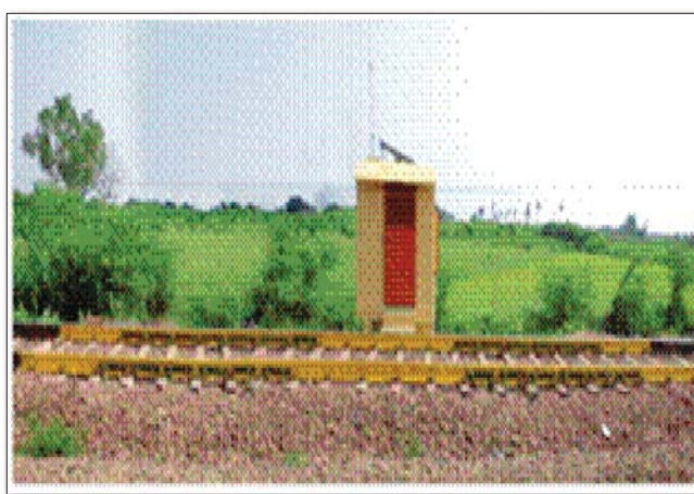
Figure 6: Wheel Impact Load Detector
