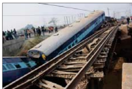
Figure 7: Train no. 12987, Ajmer-Sealdah Express derailed in Kanpur on 28.12.16
