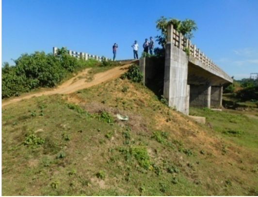
Photographs 2.3.1 & 2.3.2: (Incomplete approach road from Vitorgul end) RCC bridge over river Juri on Dharmanagar Tilthai Road to Vitorgul at Dharmanagar
