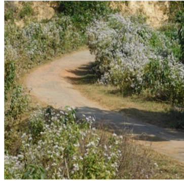
Photograph 2.5.2: At Ch: 2.1 Km
