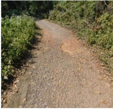
Photograph 2.5.1: At Ch: 5.5 Km
