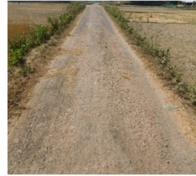
Photograph 2.5.3: Near Gamaku School
