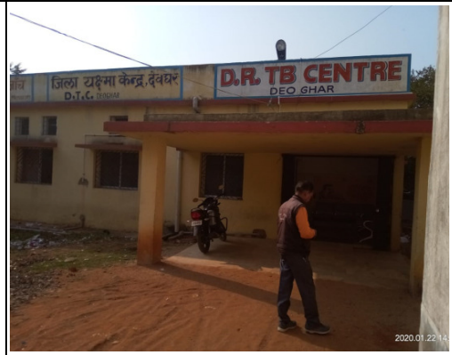
Photograph showing newly built burn unit being used as TB centre in DH, Deoghar as on 22.01.2020
