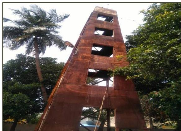
**Picture 9 : Damaged tower without ladder**
