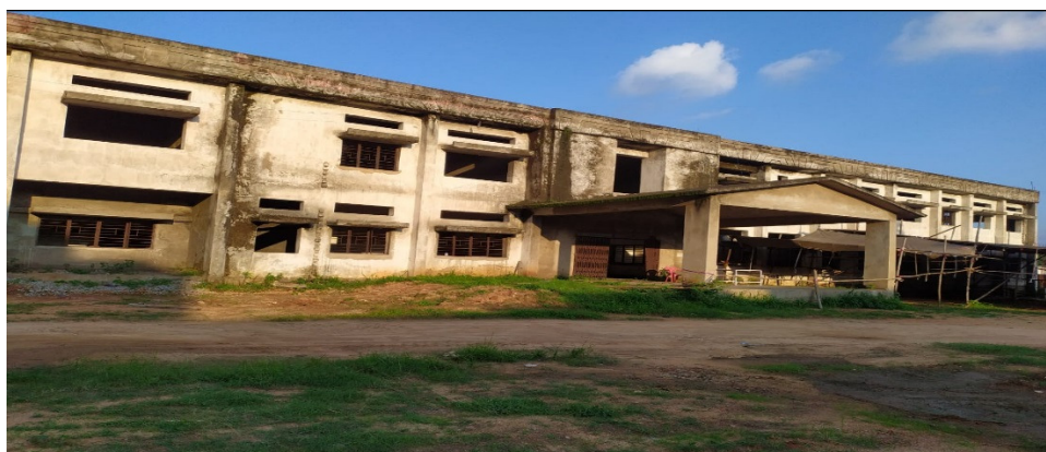
Photograph showing incomplete 100 bedded District Hospital building at Ramgarh
