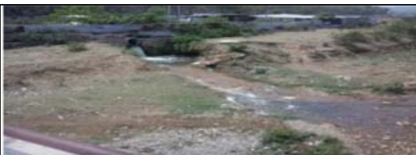
Picture No 2: Disposal of treated effluent in Nalla at Mothorowala
