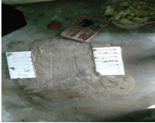
Plate 5.1: Non-functional toilet GP-Datayana, KP- Jalilpur, Bijnor, Uttar Pradesh
