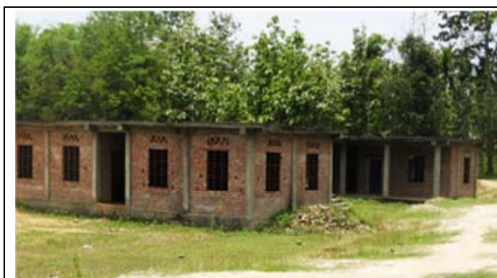
Incomplete Building- GMS Vihokhu
