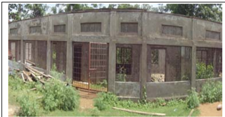
Incomplete Building- GPS Bungsang
