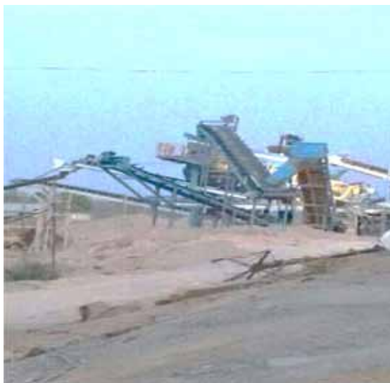
Sand crusher at site
