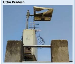
Solar panel and RCC block for bubbler was in damaged condition at Phaphamau, Allahabad at Ganga
