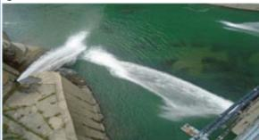
Leakage of water from the flushing conduit gates at Ichari Dam.
