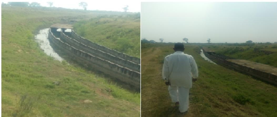
**Spillage of water between Chainage 760 and Chainage 782 during Joint Physical Verification**
