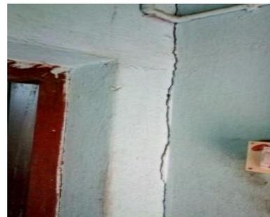
DMG and KSPCB stated that they did not have the capacity to measure the impact of vibrations due to blasts. We observed that the fixation of 100 m distance may require rethinking as functioning of quarries even at a distance of beyond 100 m caused damage to properties and created fear among the public.
