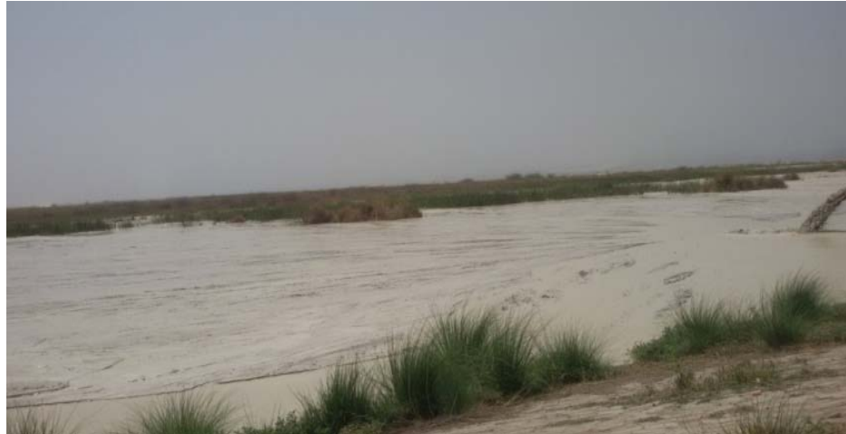
Fly-ash dump of NTPC Power Plant, Sonbhadra
