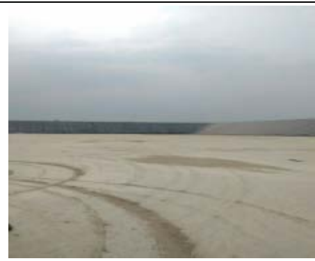
Incomplete landfill site at Shivri, Lucknow
