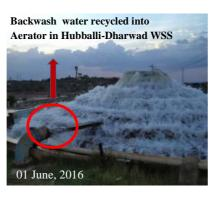
is then usually disposed of as waste water. As per the standards of the Central Pollution Control Board, the quantity of filter backwash water is normally about five *per cent* of the designed capacity of WTP. As a water conservation measure, WTPs can recycle filter backwash water so that backwash water is recovered and becomes reusable, thereby increasing the amount of treated water available and decreasing the amount of effluent.
