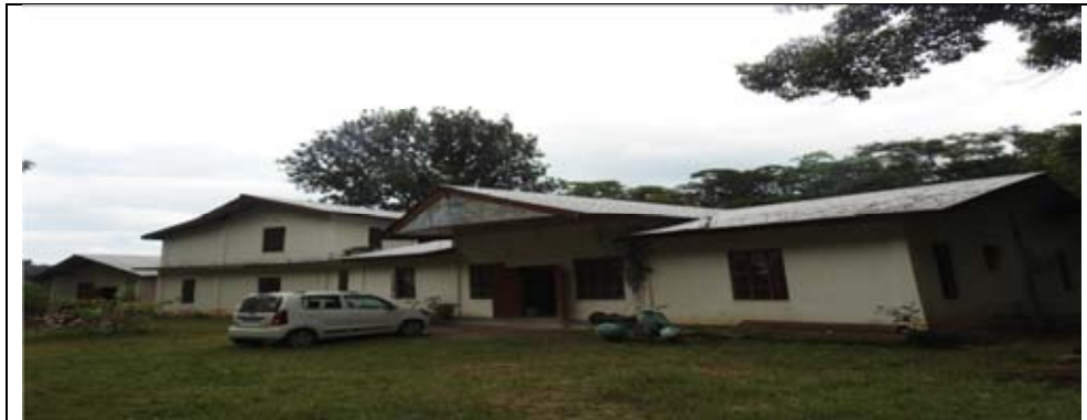
Photograph of Tourist building at Thilixu illegally occupied by land owner
