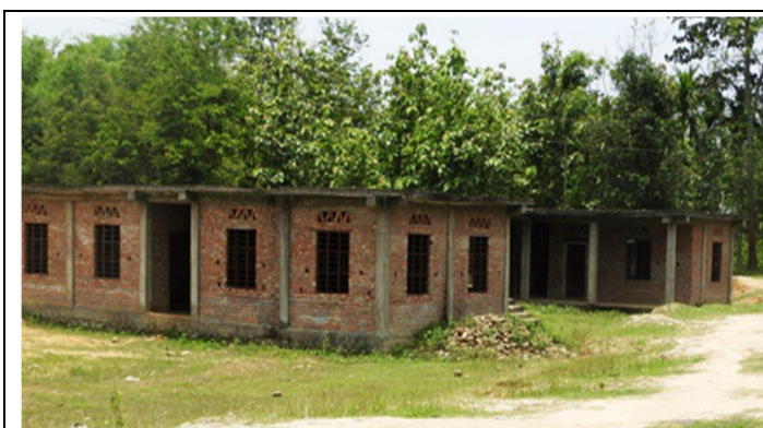
Incomplete Building- GMS Vihokhu
