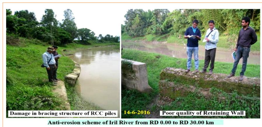
Damage in bracing structure of RCC piles
