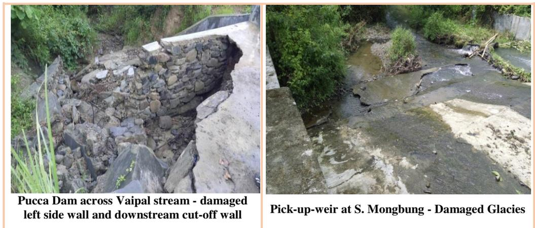
The Department stated that the damaged structures would be repaired at the earliest. During the exit conference held in November 2016, the Department stated that the damaged glaciers of Pick-up weir at S Mongbung had been repaired at the contractors cost and steps were also being taken up for early repair of other works.
