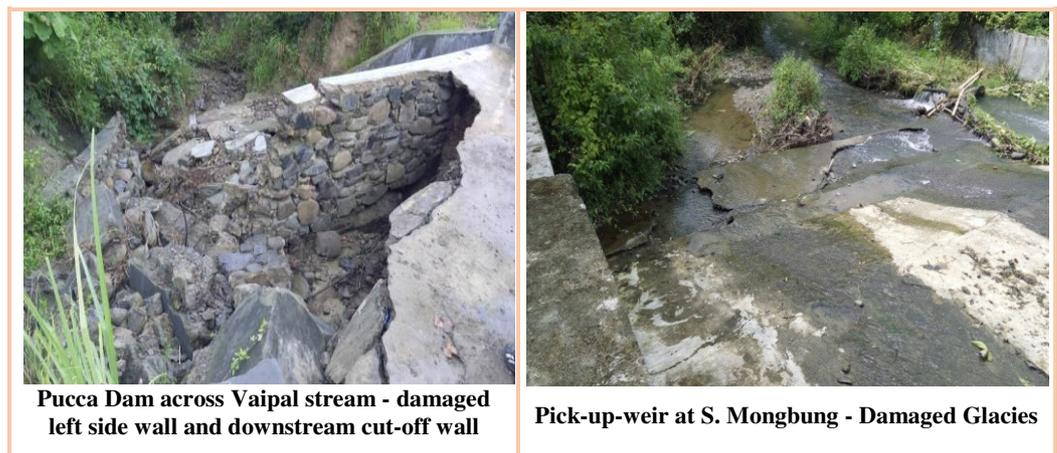
The Department stated that the damaged structures would be repaired at the earliest. During the exit conference held in November 2016, the Department stated that the damaged glacies of Pick-up weir at S Mongbung had been repaired at the contractors cost and steps were also being taken up for early repair of other works.
