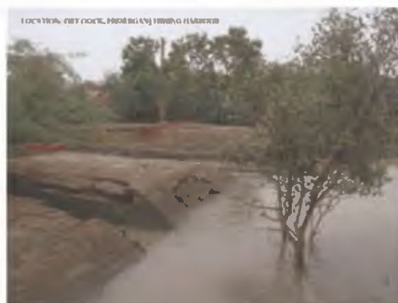
Figure : Dilapidated dry dock at Frazerganj
