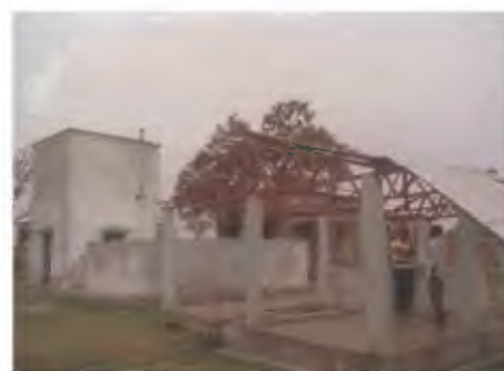
Damaged fish hatchery at Joypur
