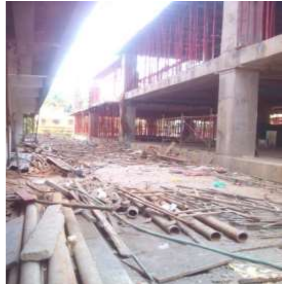
Artech shopping mall cum residential apartment at Pattoor, Thiruvananthapuram
