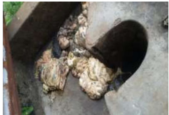
Defunct Bio-gas plant in North Paravur filled with waste
