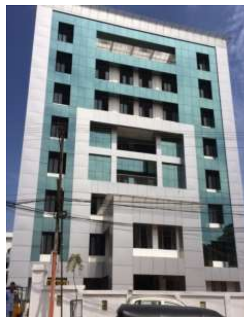
Government Secretariat – Annexe - II Building, Statue, Thiruvananthapuram
