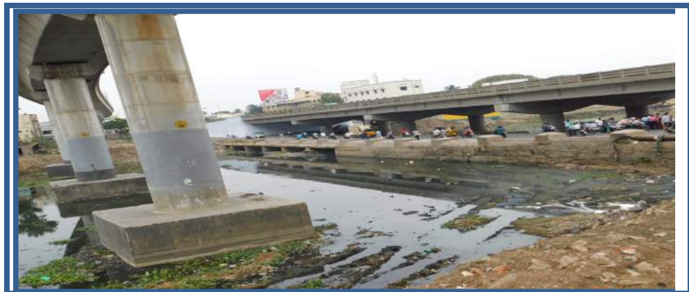
Exhibit 4.7: Metro Rail pile caps and old causeway
