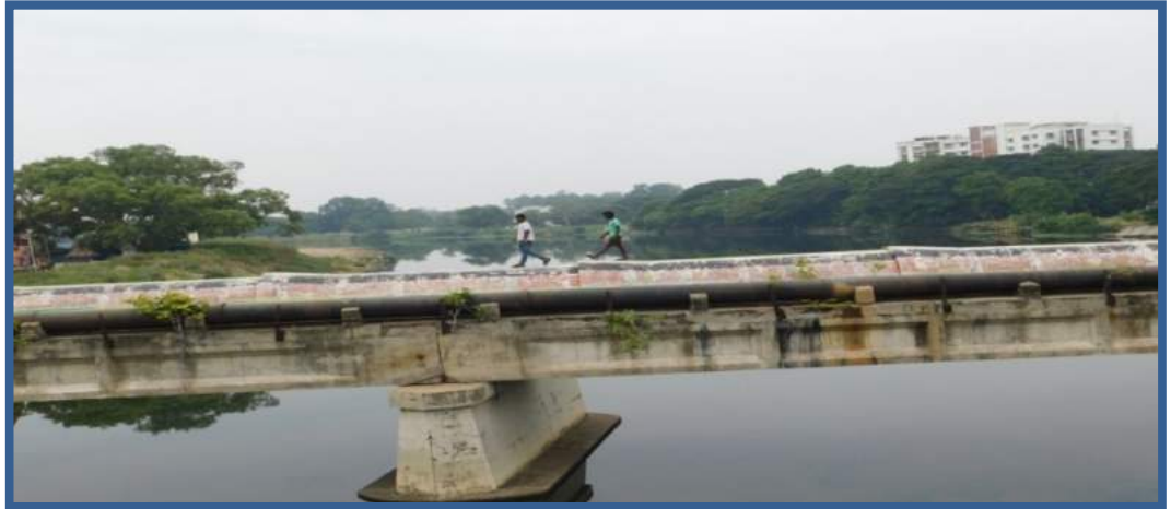
Exhibit 4.8: Old bridge blocking the free flow of water
