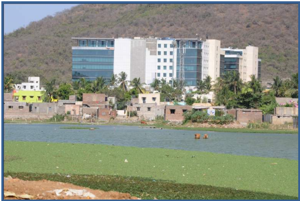
Exhibit 4.1: Encroachment in Perungalathur Big Tank
