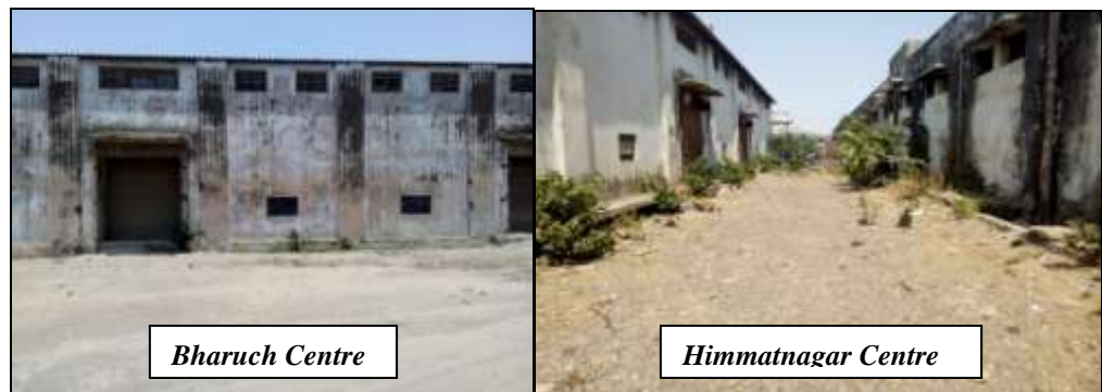
Picture 3.2: Showing poorly maintained Godowns
