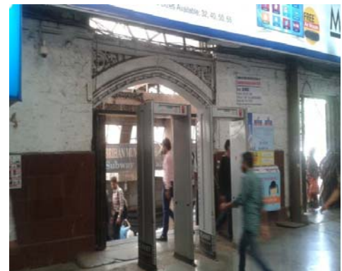
Gap at Entry/Exit point where unmanned DFMDs were provided at Mumbai CST (CR).
