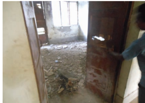
Photograph of the Hostel Building at ITI, Ambassa.
