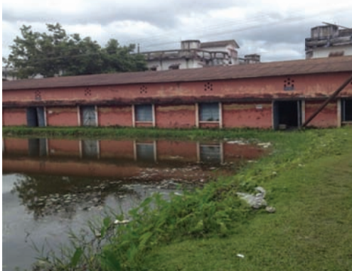
Photograph of the Workshop-cum-Class Room of the Electrician and MMV Trade at ITI, Kailashahar.
