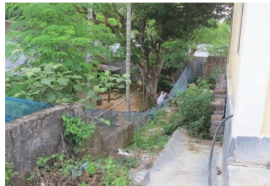
Broken compound wall of the ITI, Jatanbari in close proximity to a private household needed immediate reconstruction.
