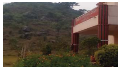
KGBV hostel building of Ch. Nuagaon without complete boundary wall
