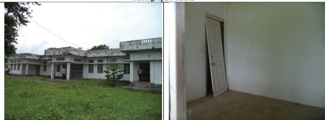
Unit Hospital constructed in September 2010 lying abandoned in poor condition
