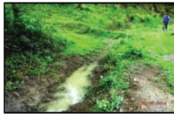
Blocked channel due to siltation and growth of vegetation
