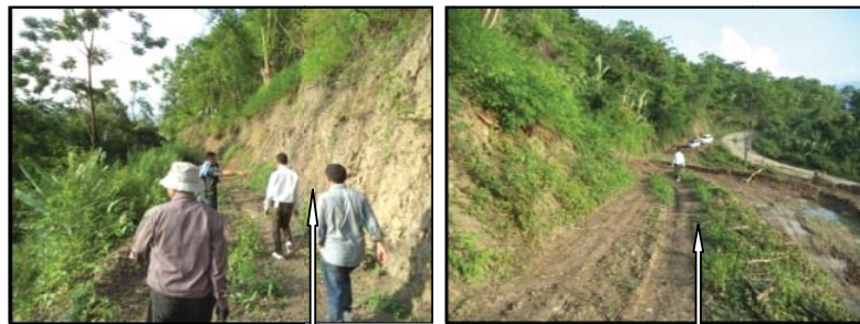
Formation cutting (approx. 2 km) for construction of lined channel
