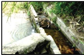
Seepage and blockage of lined channel
