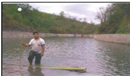
After completion of the project (September 2011)
