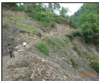
Lined channel damaged by landslide and stone crushers
