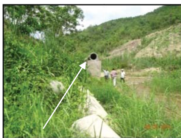
Broken hume pipe channel
