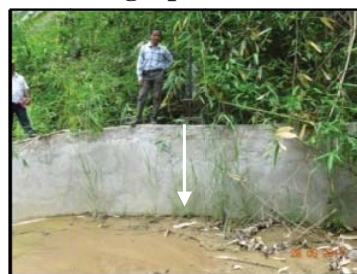
Blocked sluice due to siltation
