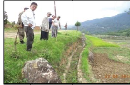
Lined channel instead of earth channel
