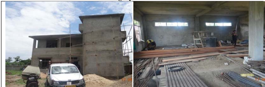
Photograph showing the ongoing construction of control room at Super Market
