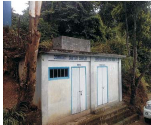
Community Sanitary Complex (Kangmun South, Lunglei District)
