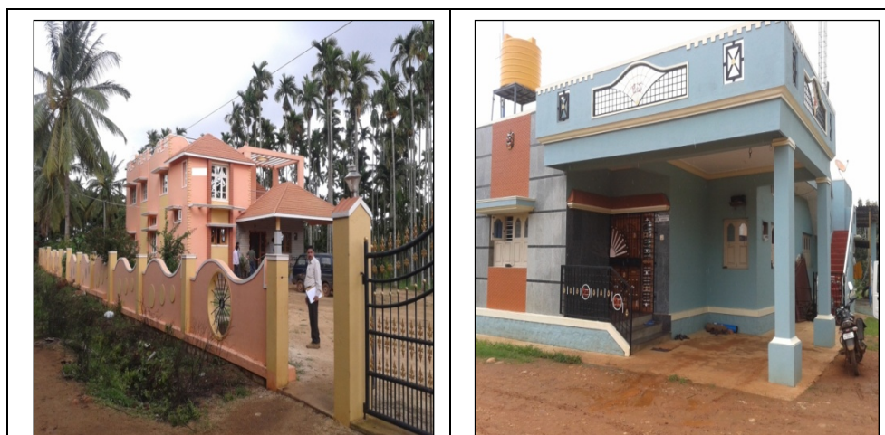
Photographs showing the houses where BPL status was doubtful (GPs, Annehal-07.08.2014 and Alagawadi-04.04.2014 of ZP, Chitradurga)
