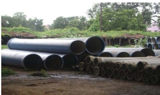
Pipes being stacked here and there without security
