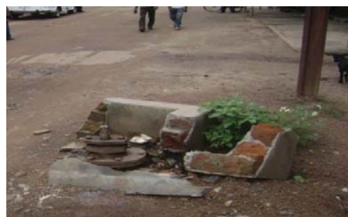
The sluice-valves are appearing above the road surface
