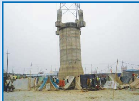
Chholdaries erected under high tension wire, Sector-6, Nagvasuki North dated 02.02.13.
