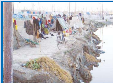
Chholdaries erected beside Mansaita Nala , Sector-12 dated 31.1.13.
