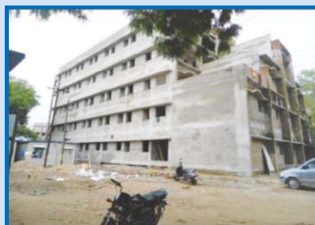
Incomplete Police Hostel on 01.09.13.
