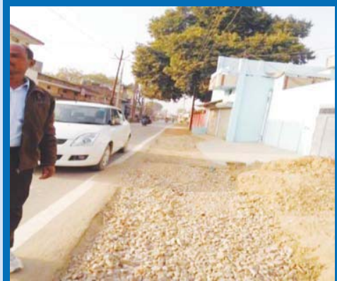
Jhansi-Allahabad-Mirzapur to Arail ghat road- interlocking/ drain work not executed as on 24.1.2013.
